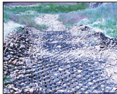
Figure 24 · Erosion control for overland discharge using rock and geotextile fabric.
