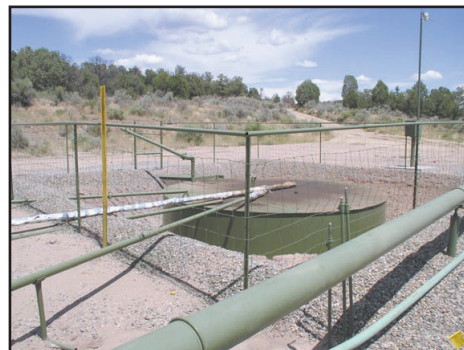
Figure 20 · A drip tank collecting condensate. The tank should be livestock and wildlife proof and should have no leaks.
