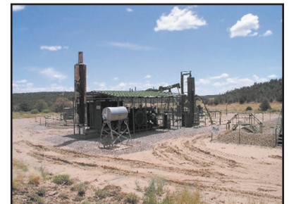
Figure 6 · CBM compressor station lacking an exterior structure and with an access road can be a source of noise pollution and traffic.
