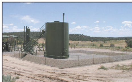
Figure 19 · A water tank is constructed atop a gravel pad with berms on all sides.
