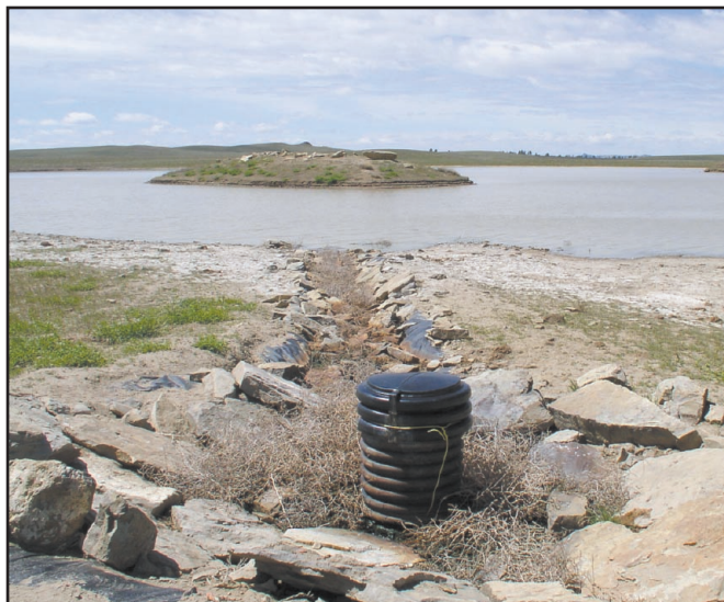
Figure 9 . CBM product water pumped from several wells is brought together to one outfall for disposal or management. This figure illustrates a CBM outfall releasing water into a constructed pond.
