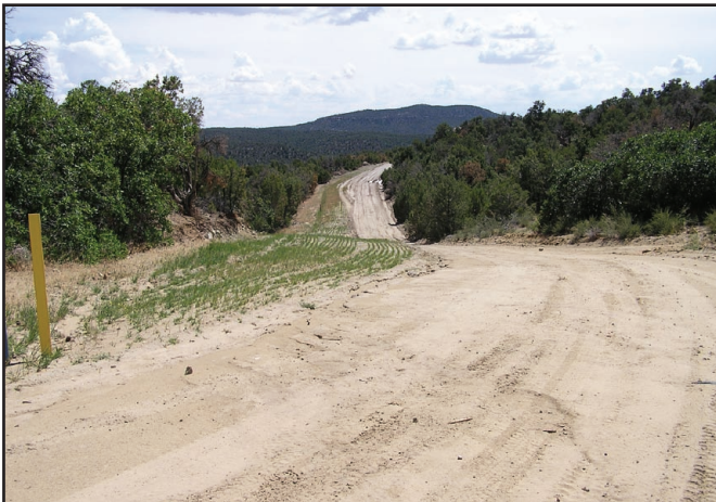
Figure 22 · Drill seeding along roadway for site stabilization and weed control.
