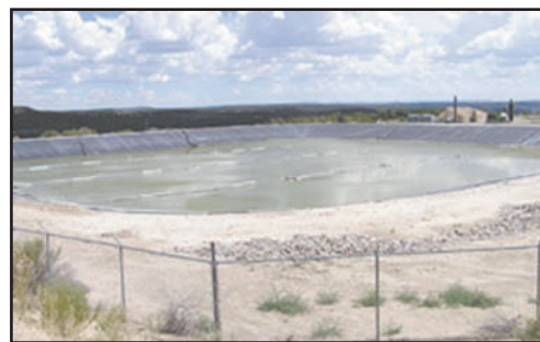
Figure 11 · Lined evaporation pond to avoid discharge of CBM water to subsurface.
