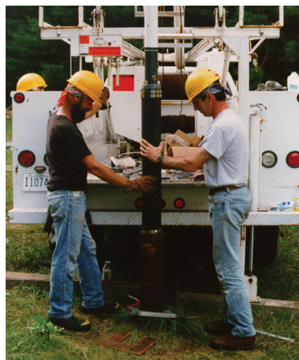
Figure 2. A borehole packer with inflatable bladder is being prepared for installation in a bedrock borehole. The packer is supported by a pipe and lowered down the borehole using a truck-mounted winch.
